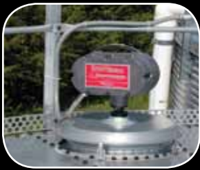
Measuring polystyrene in a polymer manufacturing facility.
